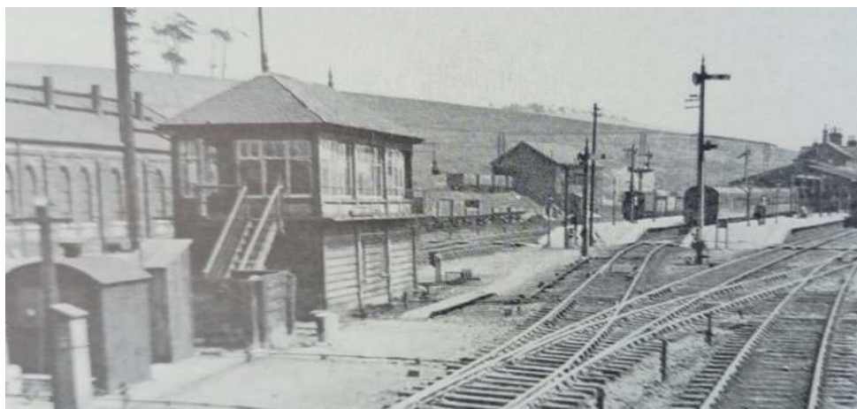
As a boy, Brian would have recognised this view of the station. Photo shows the North Box with Engine Shed at the rear.
