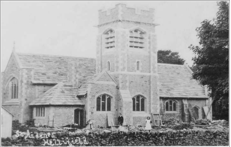
St Aidan's church under construction 1905/6
