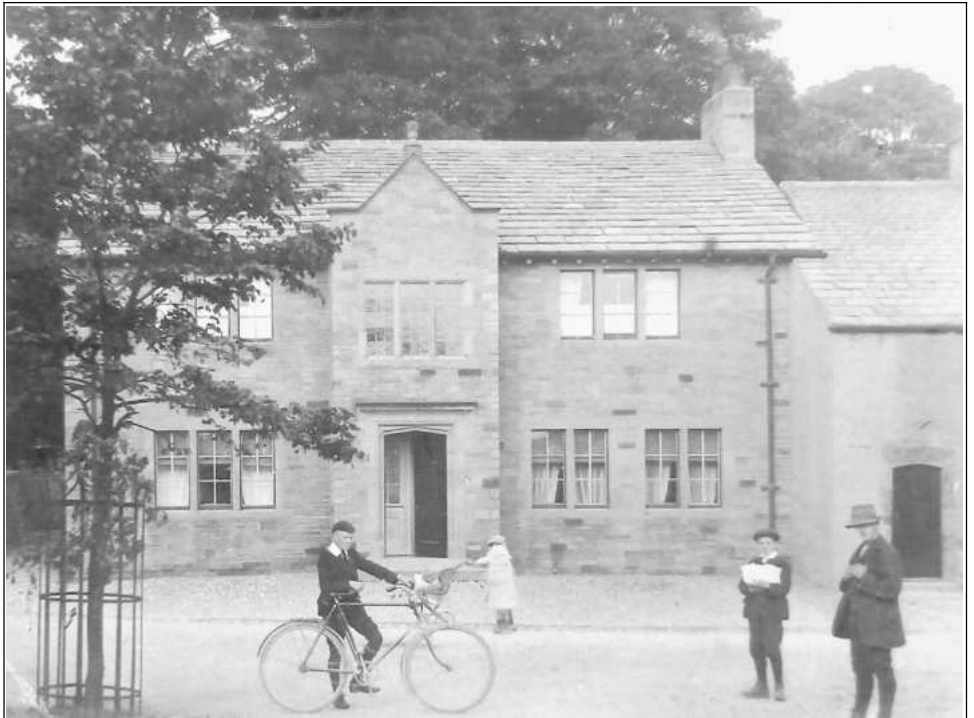
Close House. Early 20th Century. The site of Joseph Coates Butter Factor site.
